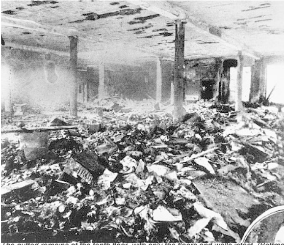
The gutted remains of the tenth floor, with only the floors and walls intact. (Bettmann/CORBIS)
