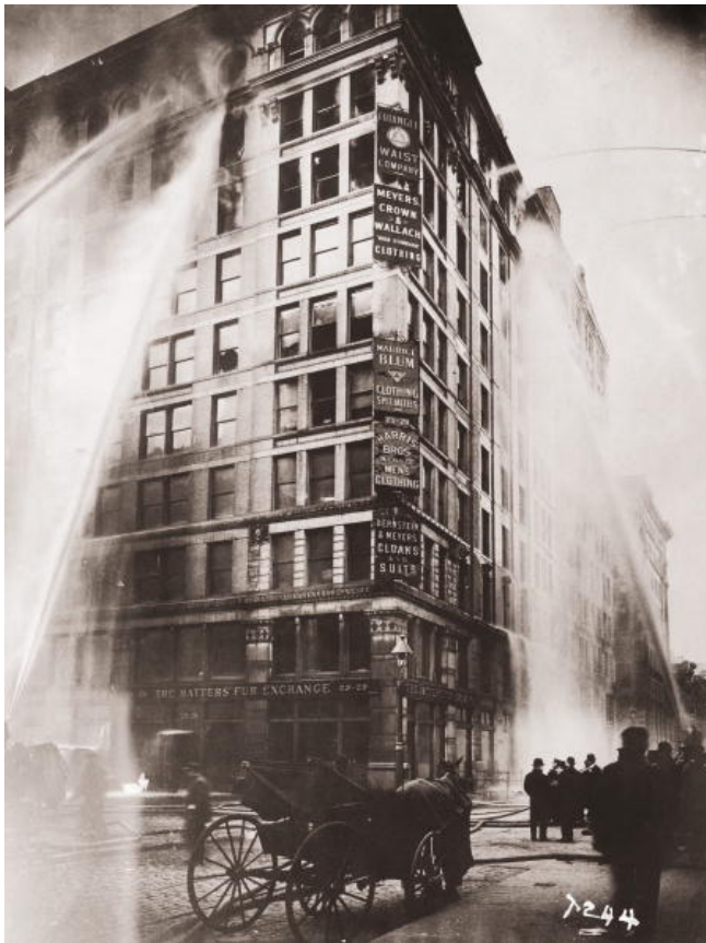
Fire hoses spray water on the upper floors of the Asch Building. (Keystone/Getty Images)
